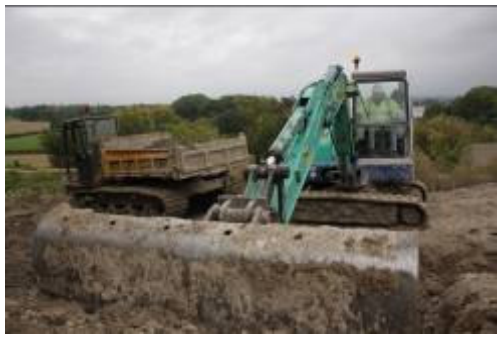
Front cover— Removing spoil for backfilling on Stage 2 Phase 2 September 2011
